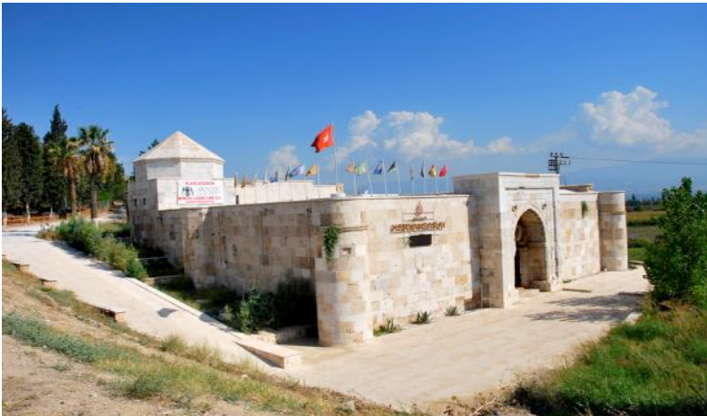
Figure 2: Akhan Caravanserai after restoration
