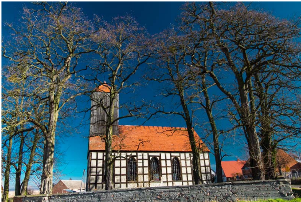
Figure 6: Church of timber frame construction, Marwice village / Western Pomerania; Source: personal picture
