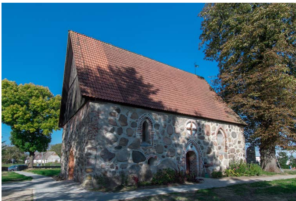
Figure 5: Medieval church built of erratic boulders – characteristic element of Western Pomeranian religious landscape; Borkowo village near Lobeż / Western Pomerania Source: personal picture
