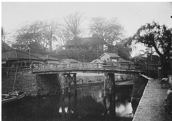
Figure 7: View of Matsuchi-yama Shoden from the Sanya Moat Source: Kitamura Photography Studio, around 1900
