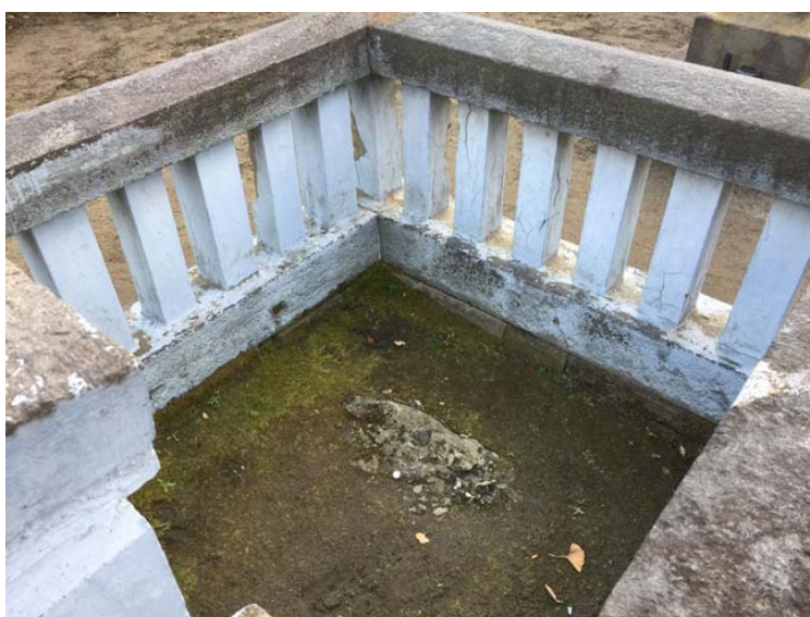
Figure 29: Top of Tateishi-sama slightly exposed from the ground.
