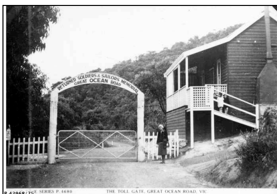
Figure 5. Memorial arch near toll gate, c. 1936 (State Library of South Australia, B43968/75).
