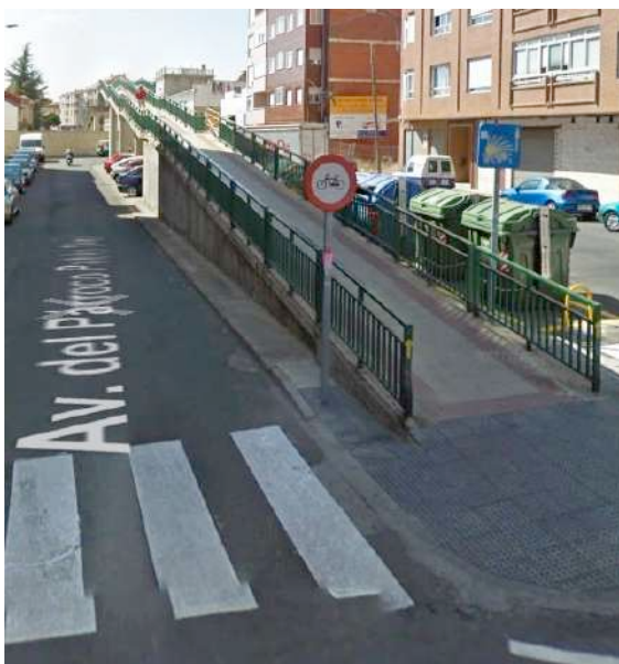
Figure 7: Access to parking in León Source: google street view
